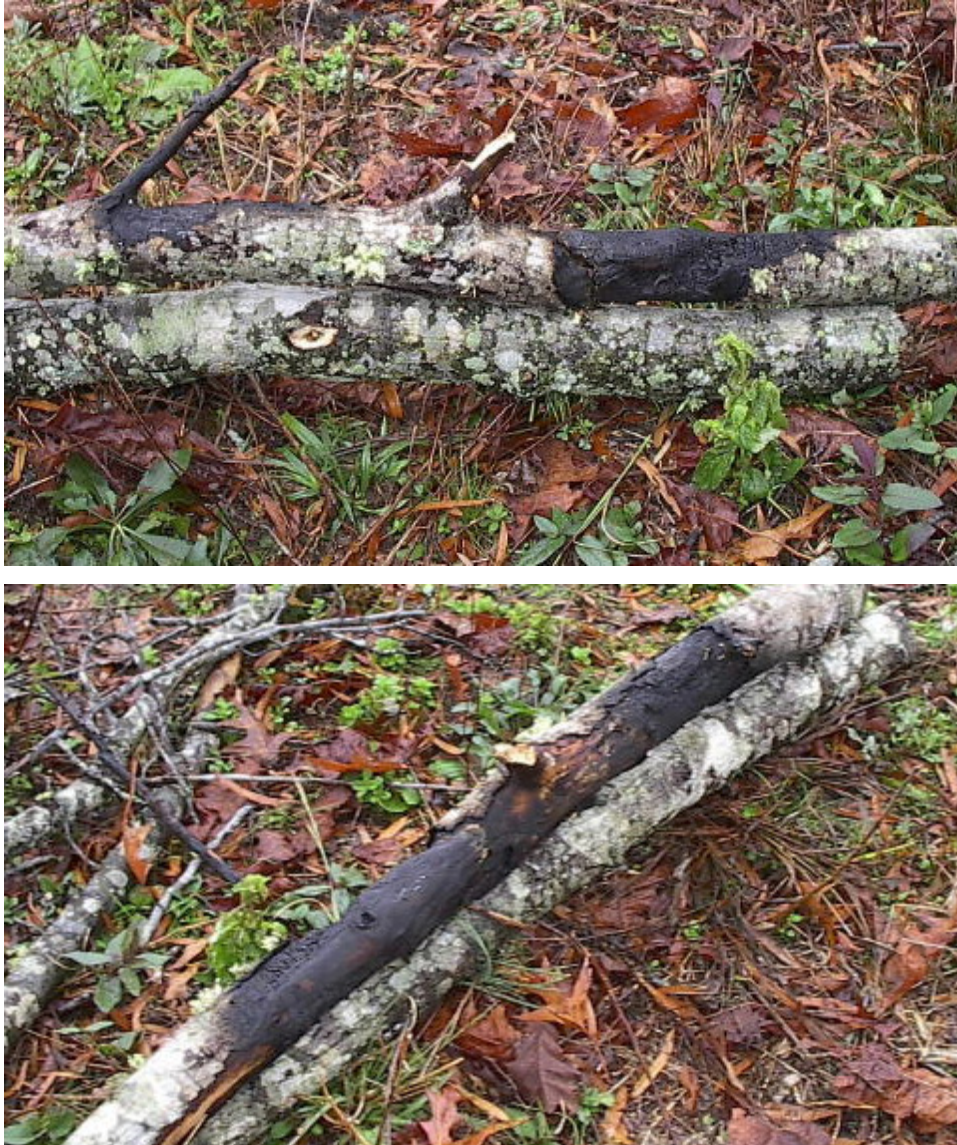
Figure 3. Tree limb tripped recloser 17 times and burned line down.
