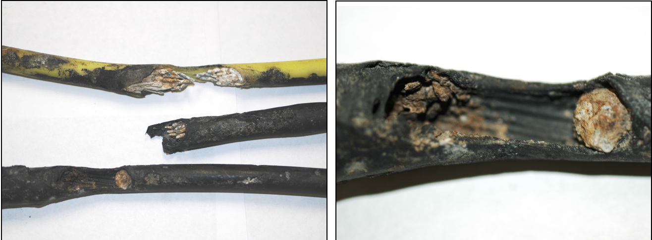
Figure 4. Excavated cables don't appear capable of serving load – but they were!
